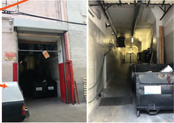
FREIGHT ELEVATOR ENTRANCE VIA ALLEY
