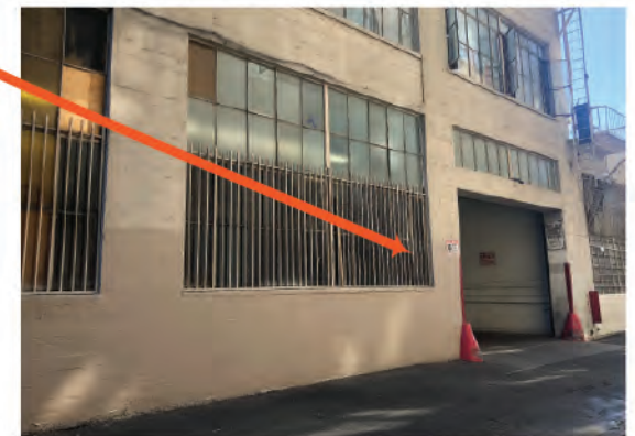
FREIGHT ELEVATOR ENTRANCE VIA ALLEY
